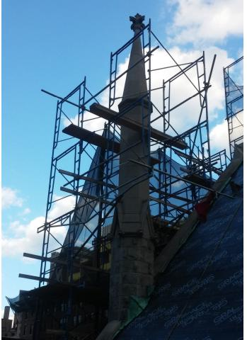
We have been referring to our project as the "Roof and Steeple Project." But it turns out to be a "Mortar Project" too. It is only sensible to do this while we have the workers and the scaffolding. The mortar work involves both the bricks and the stones in our church.
